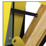
Straps keep the facades in place
